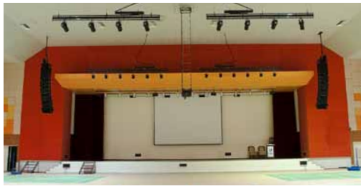
Audio System : Line array speaker, stage fill speaker, front fill speaker, monitor speaker and sub woofer
